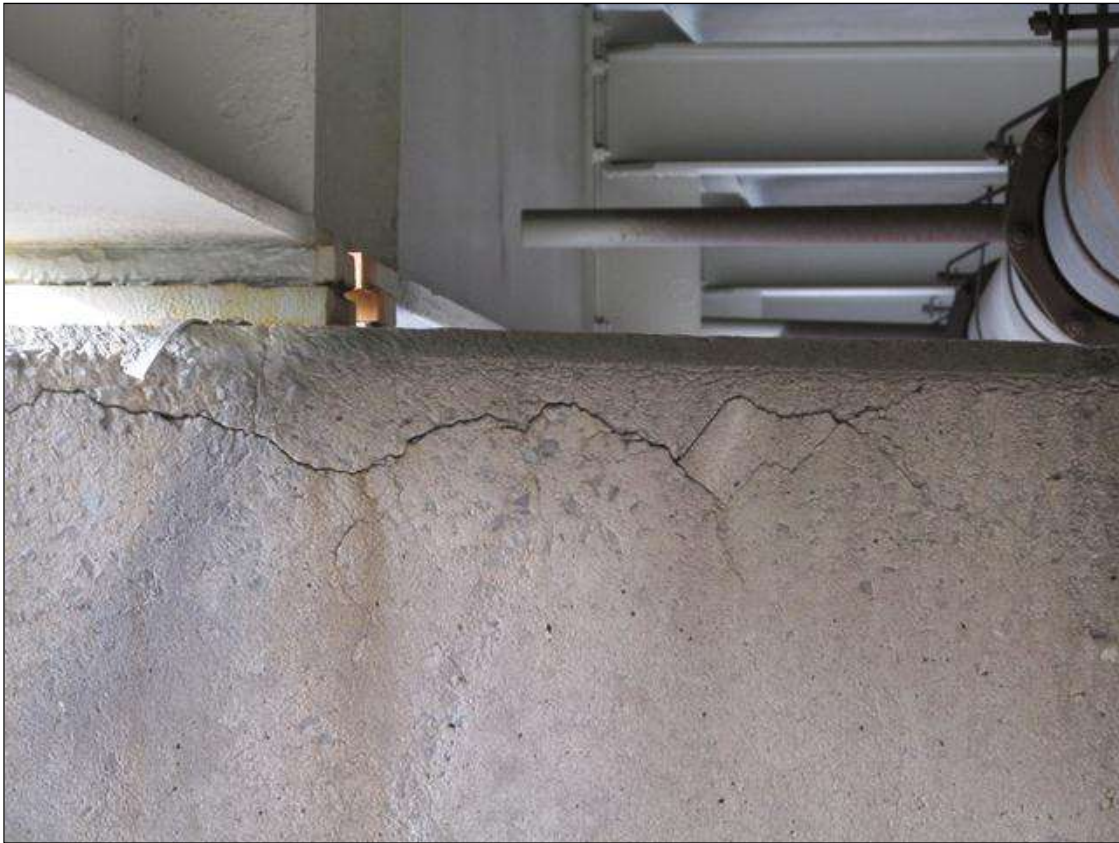
CRACKING IN BENT 3 CAP UNDER BEAMS 10-11. APPROX 8'L X 1/4"W.
