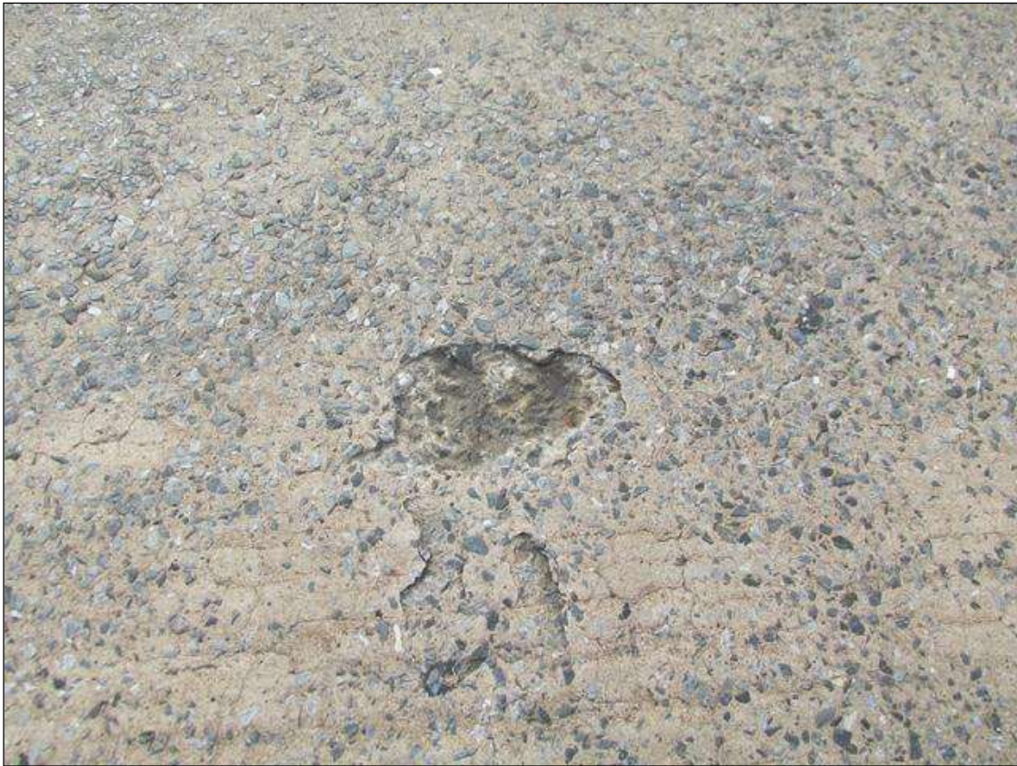
TYP SPALLING IN DECK, UP TO 1SF AREAS, SCATTERED, WITH SOME RESTEEL EXPOSED.
