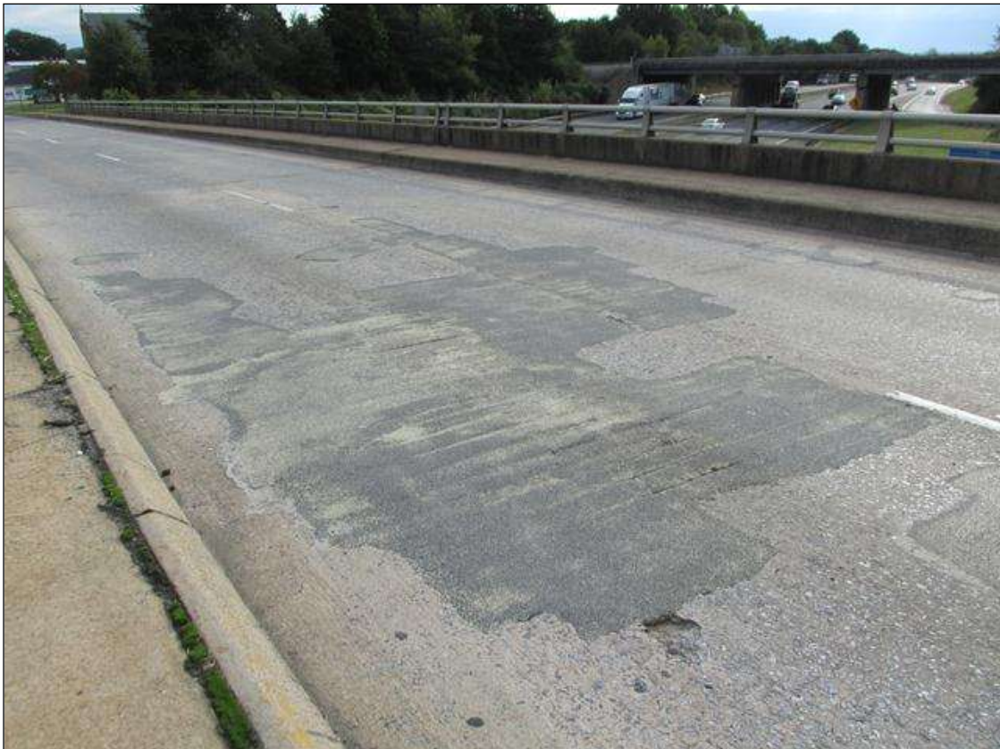
TEMP REPAIRS TO CONCRETE DECK, SCATTERED THROUGHOUT ALL SPANS AND ALL LANES. PATCHES UP TO APPROX 64SF IN SIZE.
