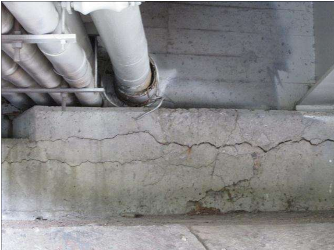
CRACKING IN ABUT 2 CAP UNDER BEAMS 1-2. APPROX 12'L X 1/4"W.
