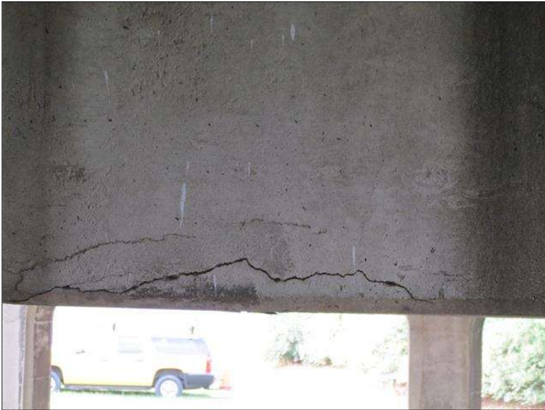
CRACKING IN BENT 3, BOTTOM SIDE OF CAP BETWEEN PILES 1-2, APPROX 8'L X 1/4"W.
