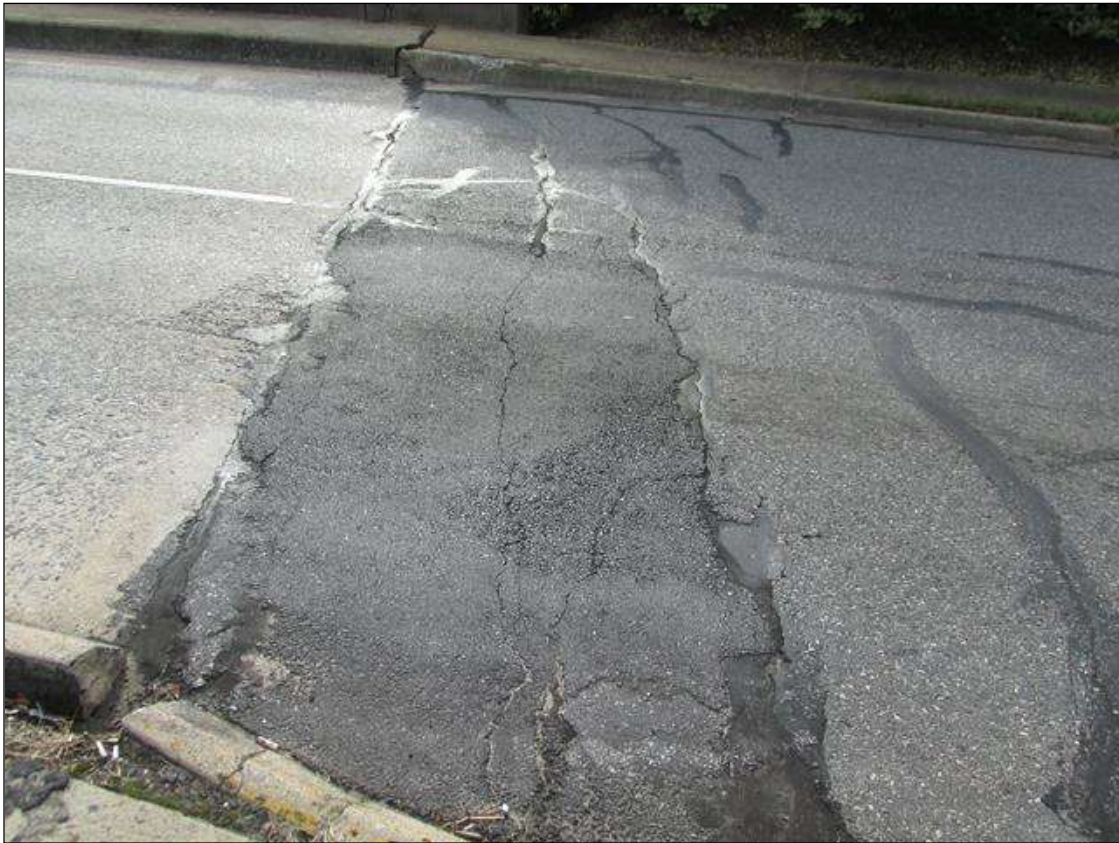
WEST APPROACH ROADWAY CRACKED AND SUNKEN UP TO 1", 20'W X 5'L
