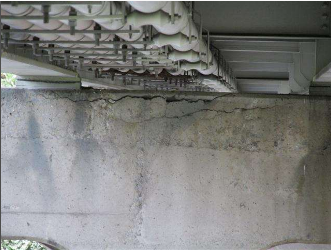
CRACKING IN RC CAP, BENT 1, BAY 1, APPROX 8'L X 1/4"W.
