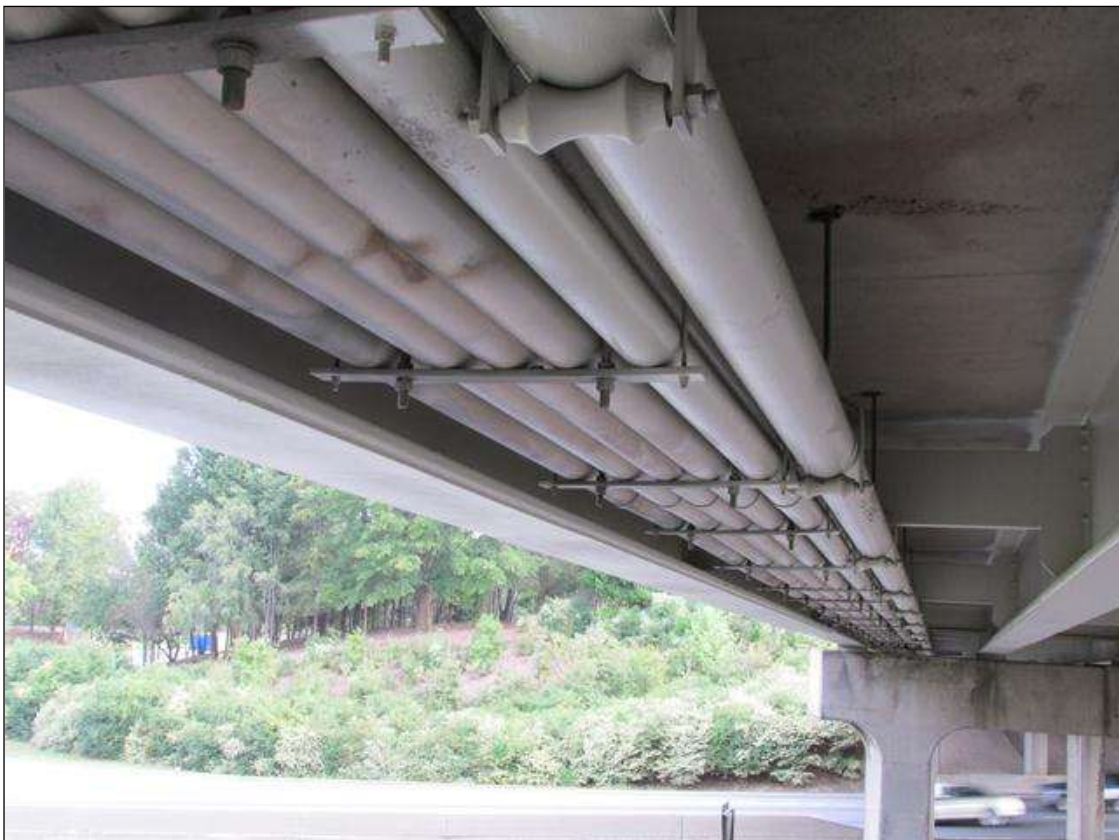
GANGED CONDUITS HANGING FROM STEEL SUPPORTS, BAY 1
