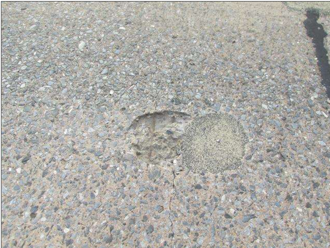
SPALLING WITH RESTEEL EXPOSED, -L- RT, INSIDE LANE, SPAN 2. APPROX 1SF AREA.
