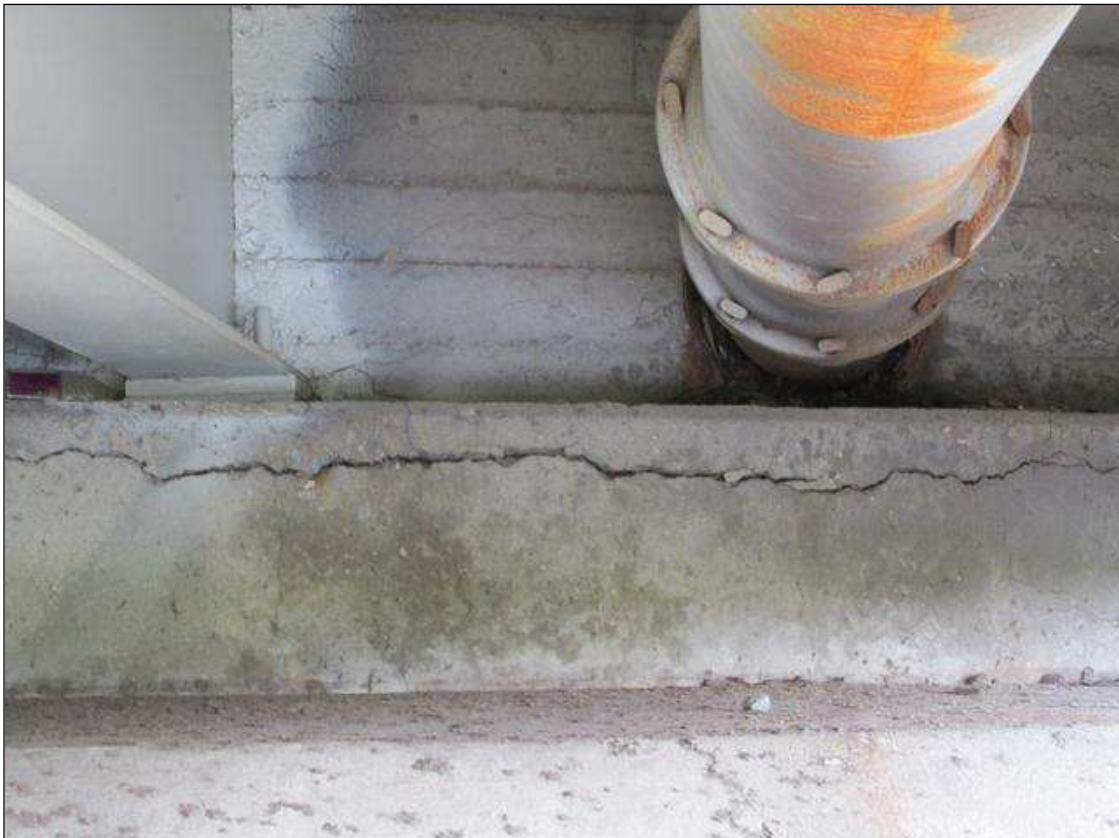
CRACKING IN ABUT 2 CAP UNDER BEAMS 10-11. APPROX 10'L X 1/4"W.
