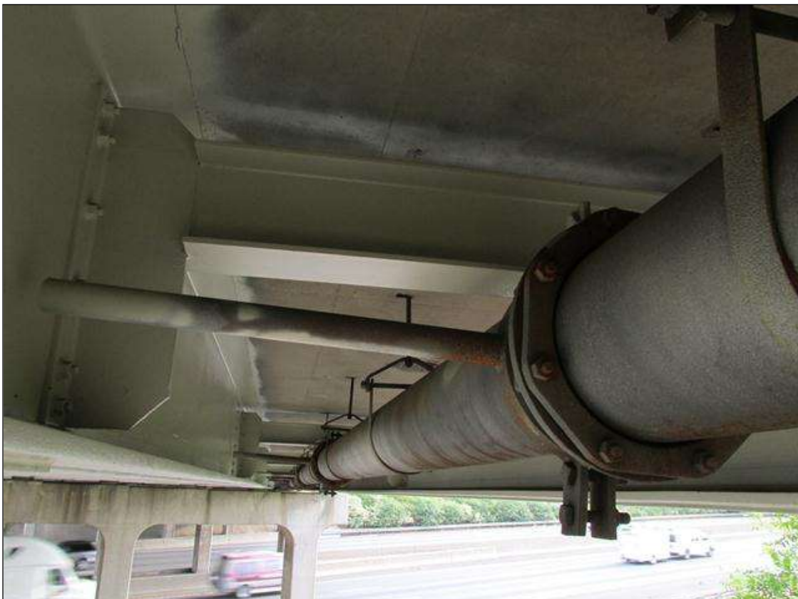
12" DIP HANGING FROM STEEL SUPPORTS, BAY 10
