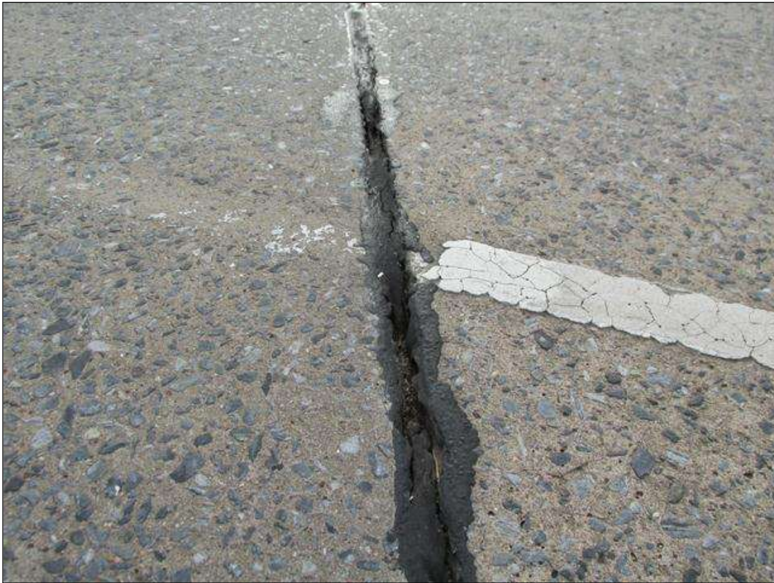
JOINT SEAL AT EAST APPROACH CRACKED WITH SECTIONS MISSING. APPROX 10' OF LOSS. REMAINING 10' IS LOOSE.
