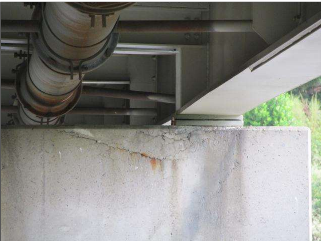
CRACKING IN RC CAP, BENT 1, BAY 10, APPROX 6'L X 1/4"W
